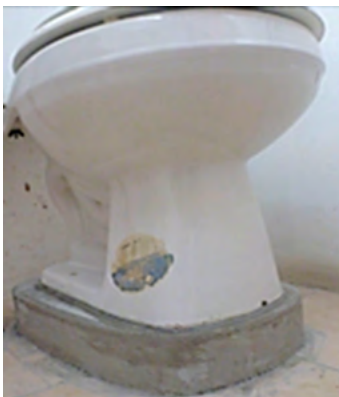
Photo 7: Raised toilet seat with concrete base
